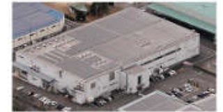
Japan (Toyohama Manufacturing Site)
